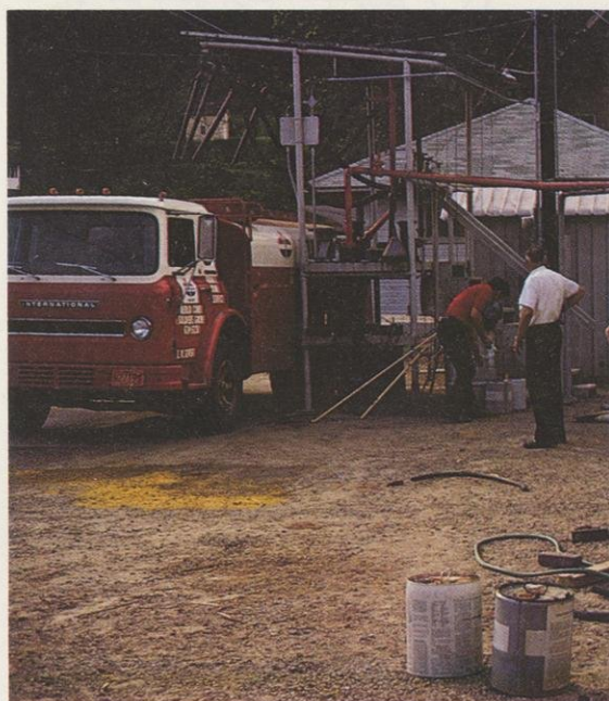
In the early 70's, pesticides were accidentally siphoned into a community system from a supplier's tank when pressure in the system dropped after it was shut down for repair. The contaminant was quickly discovered and flushed out. DNR photo
