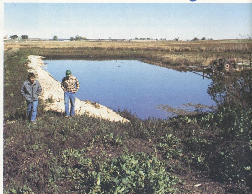
Wastes from processing plants are disposed of in lagoons or by spray irrigation. Both are carefully regulated by DNR to prevent harm to surface and groundwater. Photo by Dean Tvedt
