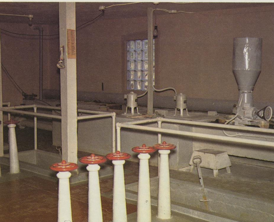
DNR continually tests the state's 1,300 community water systems for toxics and other contaminants. These are operating controls for a filter system. DNR photo
