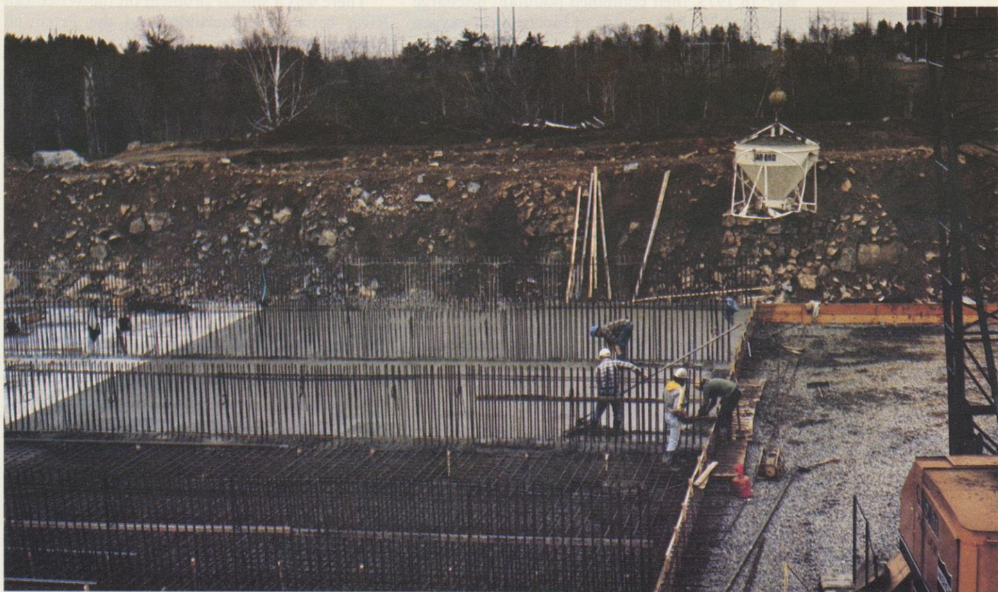
Pouring concrete for the primary clarifier at the new $11.7-million Rib Mountain wastewater treatment plant. DNR contributed $7-million to the project. Photo by Jerry Neis
