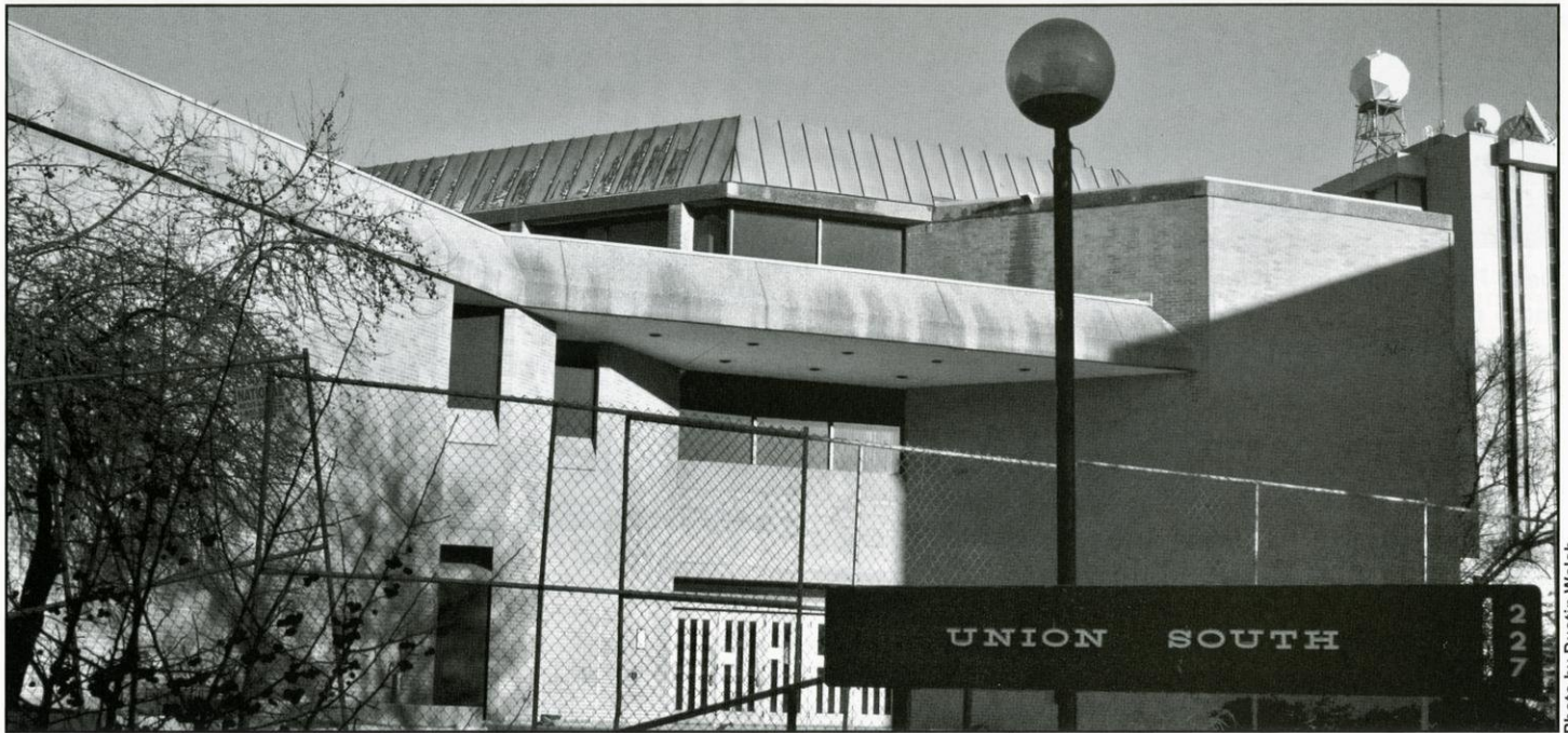
Fences surrounding Union South force pedestrians to find new walking routes.
