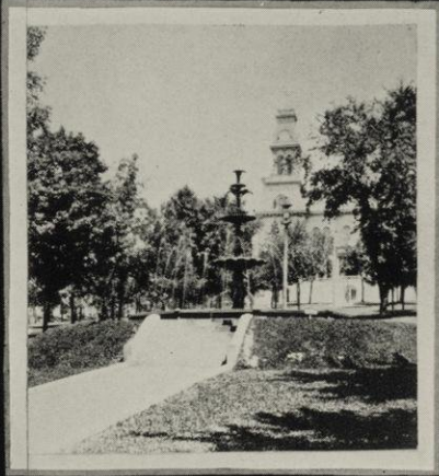
Notice the Lighting System
