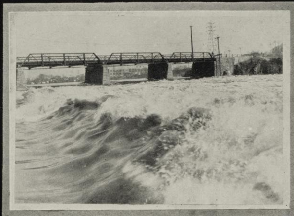
A later bridge at Monterey
