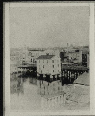
View North West Milwaukee St. Bridge
