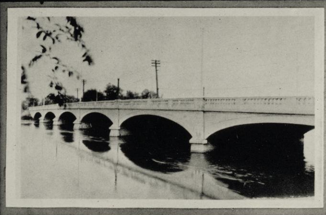
Jackson St. Bridge
