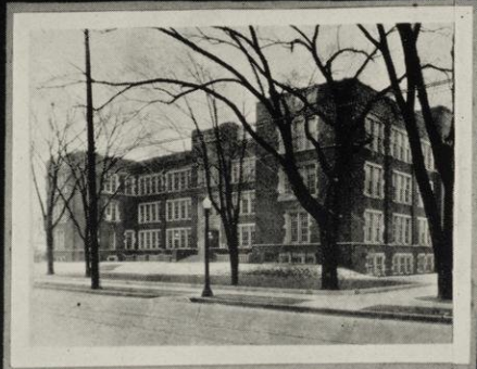
High School 1935. Corner stone laid 1921
