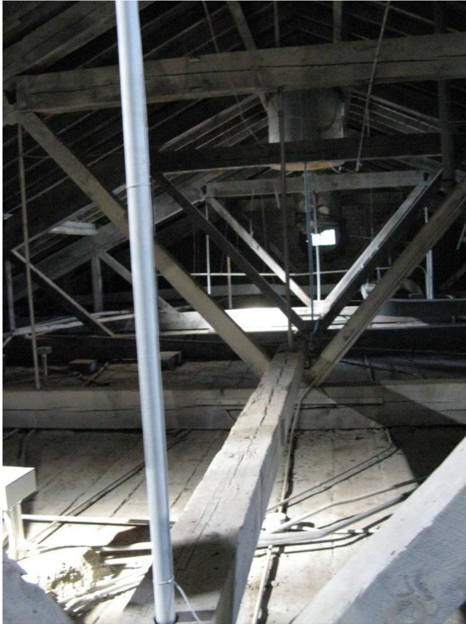
Figure 2.26. The framing of the roof of the Center Main. The roofs of the Flats were constructed with the same materials. (Photo by the author, 2007)
