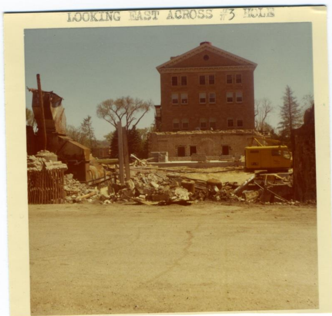
Figure 4.2. The Old Main next to the demolition of the Flats, 1967. (Photo courtesy of the St. Peter Regional Treatment Center Museum).
