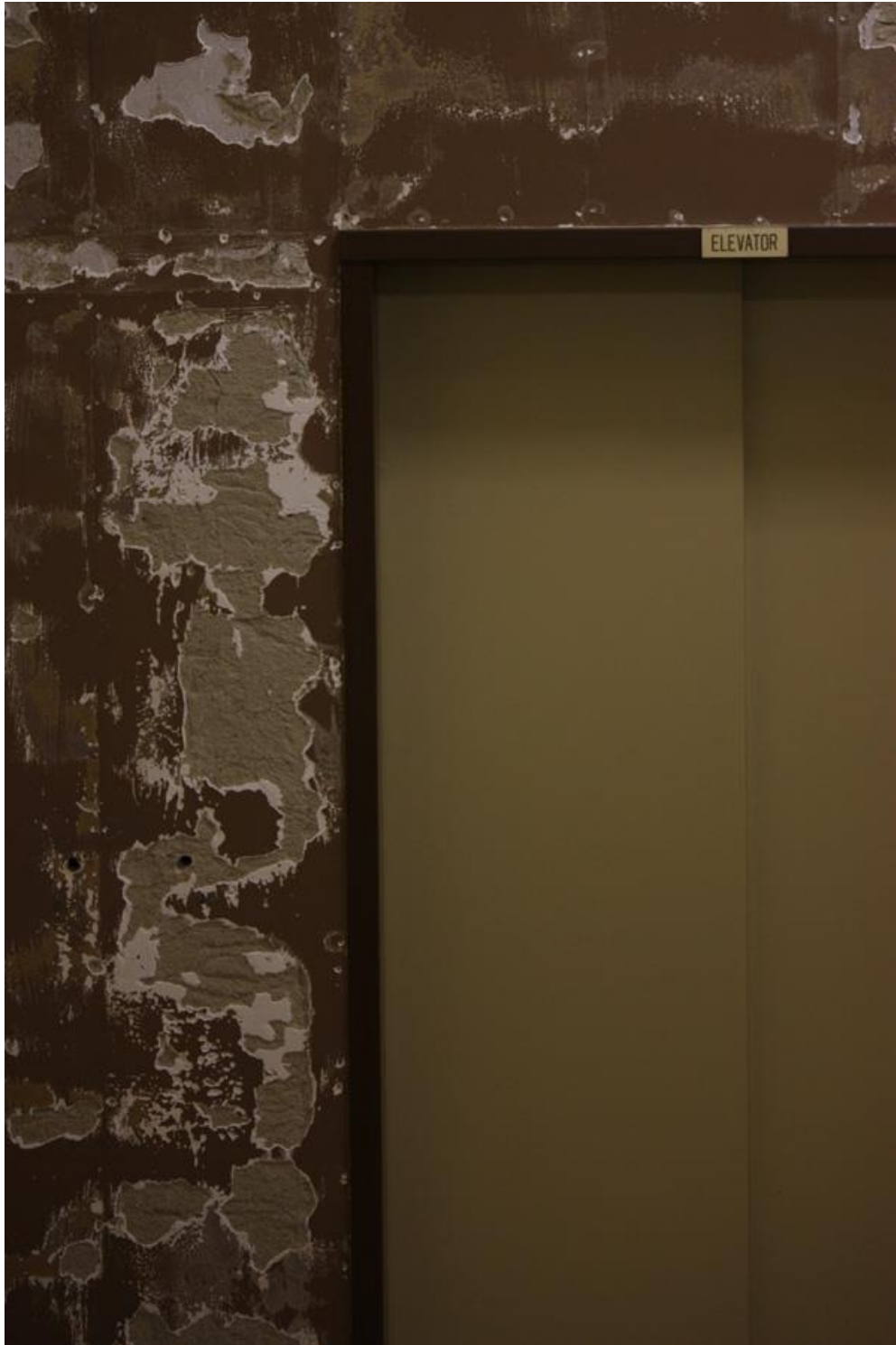
Figure 4.4. The Otis elevator at the SPRTC. (Photograph by author, 2010).
