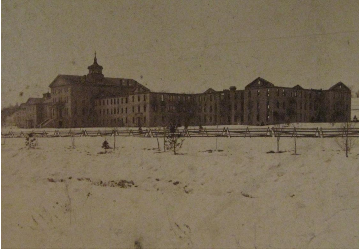
Figure 2.25. The hospital, from the north-east, 1880. You can see how the shell of the building remains while the roof and the interior have been burned away.
