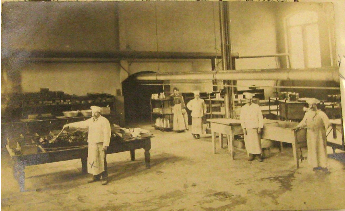
Figure 2.23. Main Kitchen in the basement of Center Main. The large black doorway in the back of the room leads into the tunnels. (Image courtesy of the University Archives at Minnesota State University, Mankato.)
