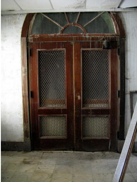
Figure 2.17. The door in Old Main that once led to the southern ward, also known as South Flat. The false ceiling can be seen cutting off the top of the window. (Photo by the author, 2007)
