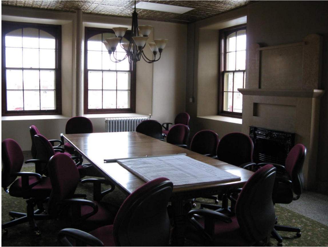
Figure 2.21. Originally the parlor for visitors, this room has been remodeled in 2008 to serve as a meeting room. The false ceiling is newly installed and conceals a ceiling of at least two feet more in height. (Photo by the author, 2008)
