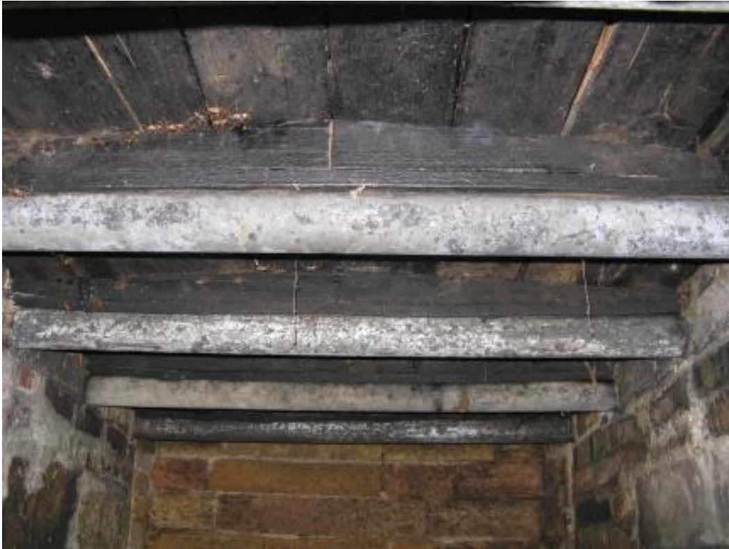
Figure 3.21. Ceiling/roof support inside Earl's shack (Photo by the author, 2010).
