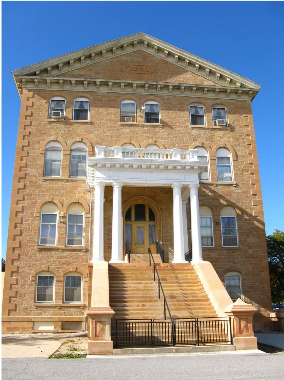
Figure 4.8. Door (Outside) in the SPRTC Museum that used to be an entrance to the library. (Photograph by author, 2010).
