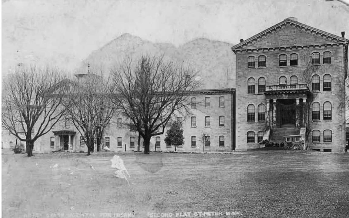
Figure 2.27. Separation of Flats from Main, circa 1910 (Photo courtesy of the St. Peter Regional Treatment Center Museum Collection)
