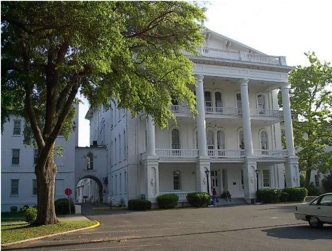
Figure 2.8. Alabama Hospital for the Insane at Tuscaloosa, date unknown.
