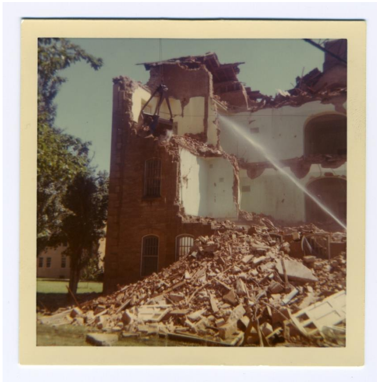
Figure 4.1. Demolition of the South Flat, 1967. (Photo courtesy of the St. Peter Regional Treatment Center Museum).
