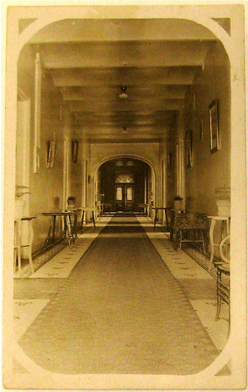
Figure 2.30. Lower Flat North, looking south, toward the doorway to Old Main. Date unknown. (Image courtesy of the University Archives at Minnesota State University, Mankato.)
