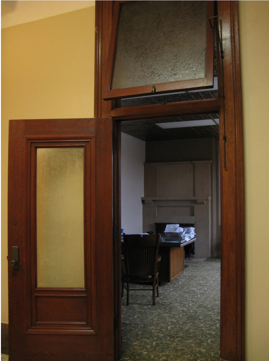
Figure 2.20. Originally the superintendents office, this room has been remodeled in 2008 to serve as office space for administration. The wall on the left side of the room was a previous addition, but it is unknown in what year it was put up. The door, doorframe, and glass panes are original. (Photo by the author, 2008)
