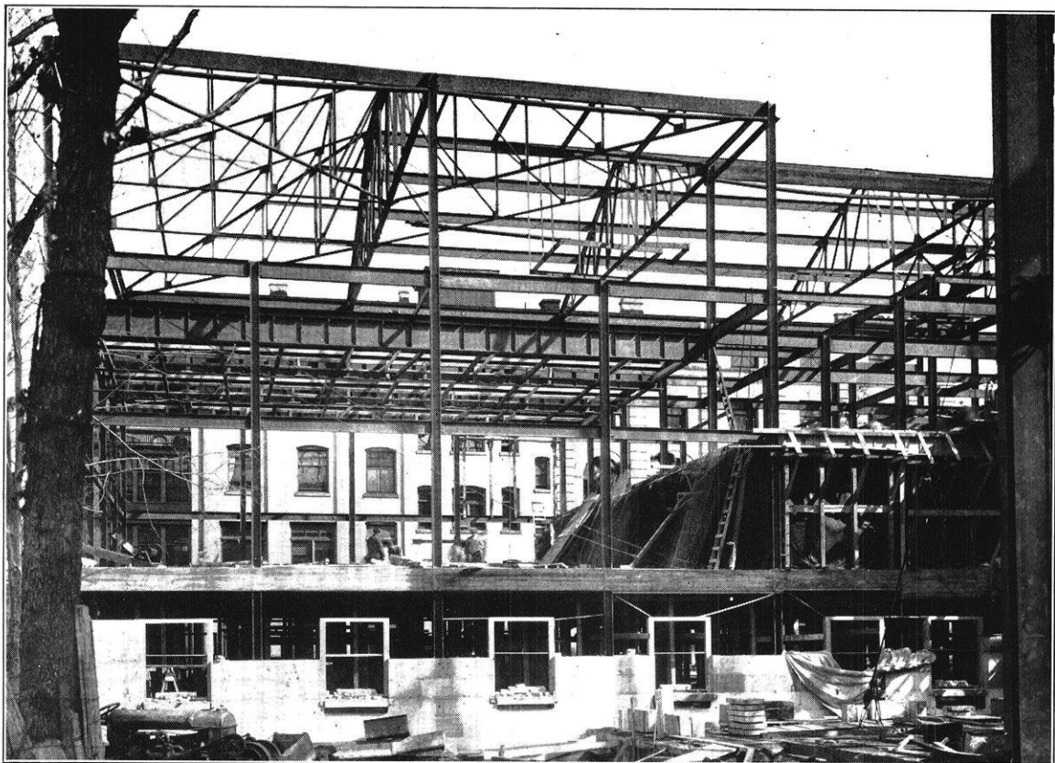
DETAIL OF MEMORIAL UNION STEEL — TRIPP COMMONS
