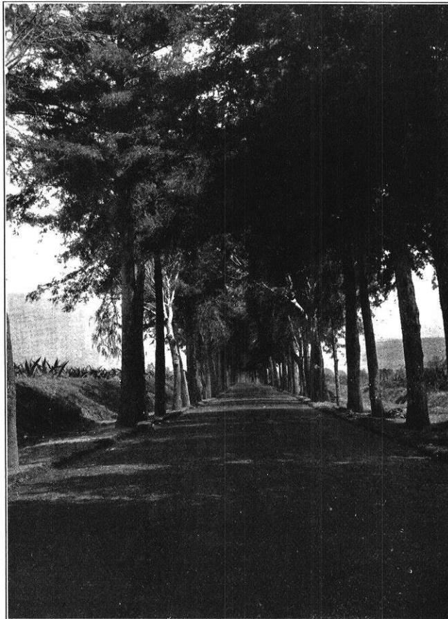
Completed Oil-treated Road
