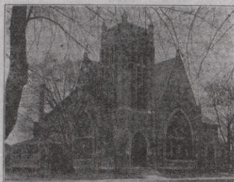
Corner of Church Street and Columbia Avenue Church Floor 64
