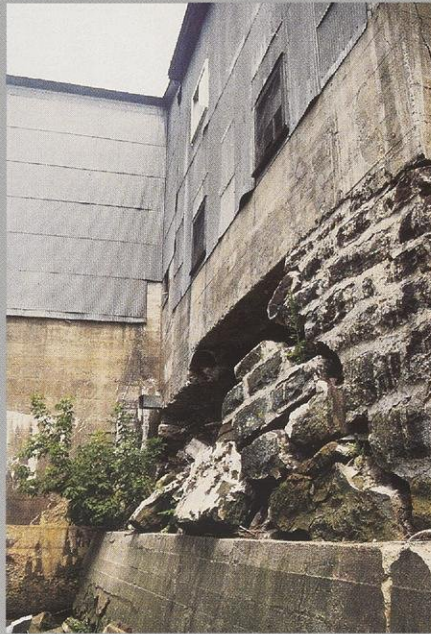
Deteriorating masonry at a dam. Of Wisconsin's 3,600 dams, fewer than 200 generate electricity and only 30 percent must be inspected once a decade.
