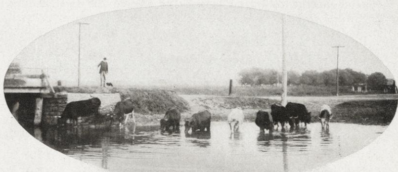
Site of Steensland Bridge, 1897
