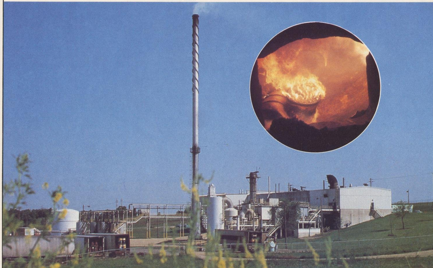
This 3M incinerator, located east of St. Paul in Minnesota is especially designed to handle 55 gallon drums. It burns at temperatures up to 2200 degrees fahrenheit and includes both air and water pollution control equipment. Photo courtesy of 3M Corporation
