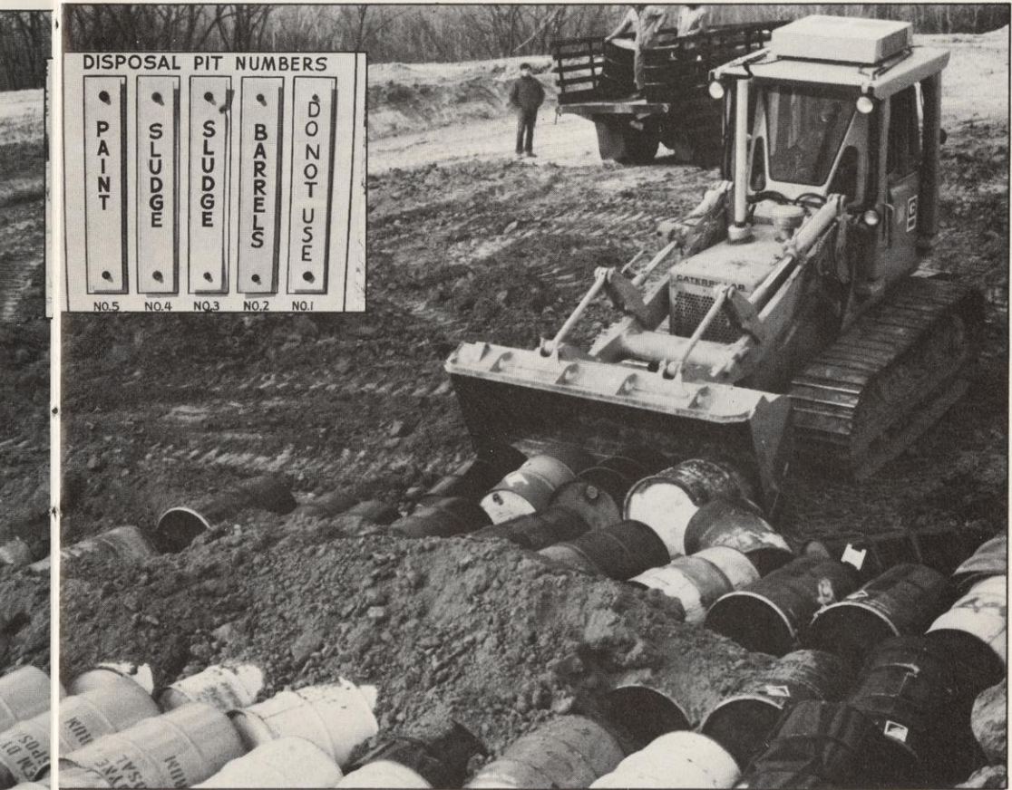
Safely buried, barrels are sealed in clay, which prevents underground migration of the materials they contain. Photo courtesy of EPA
