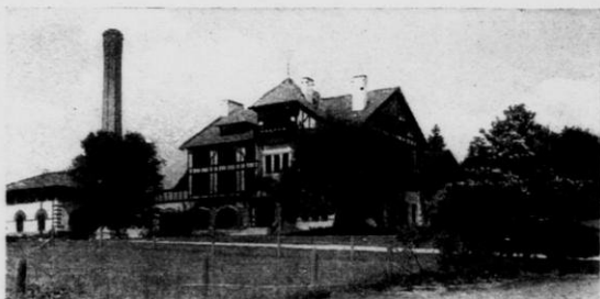
The Dairy Building
