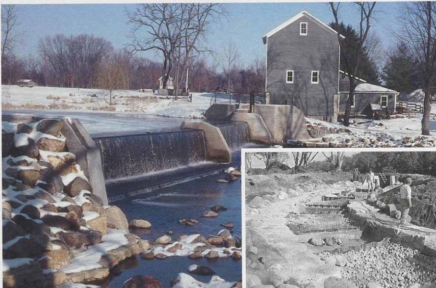
Beckman's Dam on the Rock River in Green County is the site of a recent fishway success story. The fishway gradually sweeps off the bottom left side of this photo up shallow steps.
