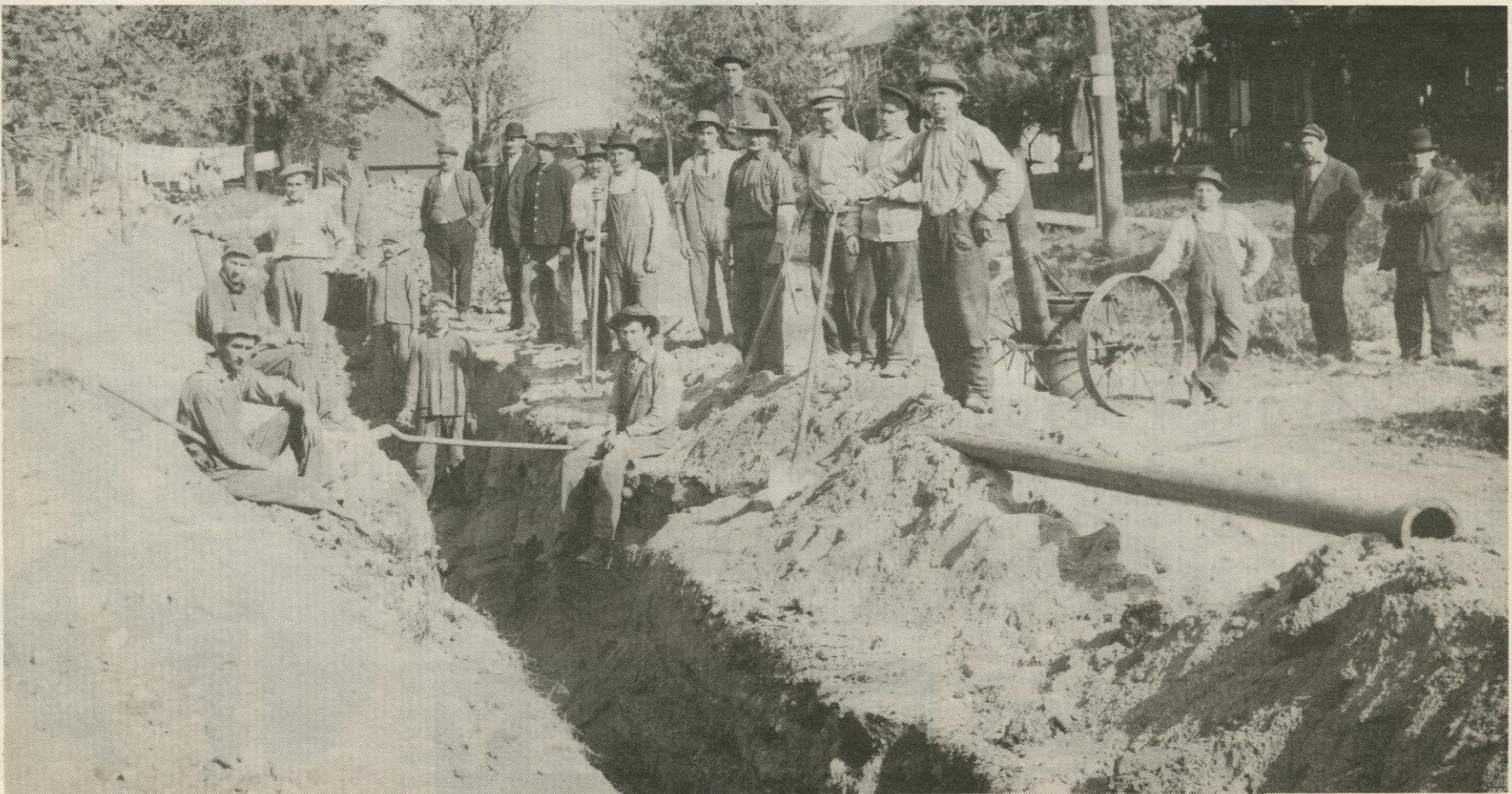
Installing sewer, water and gas lines in Fort Atkinson.
