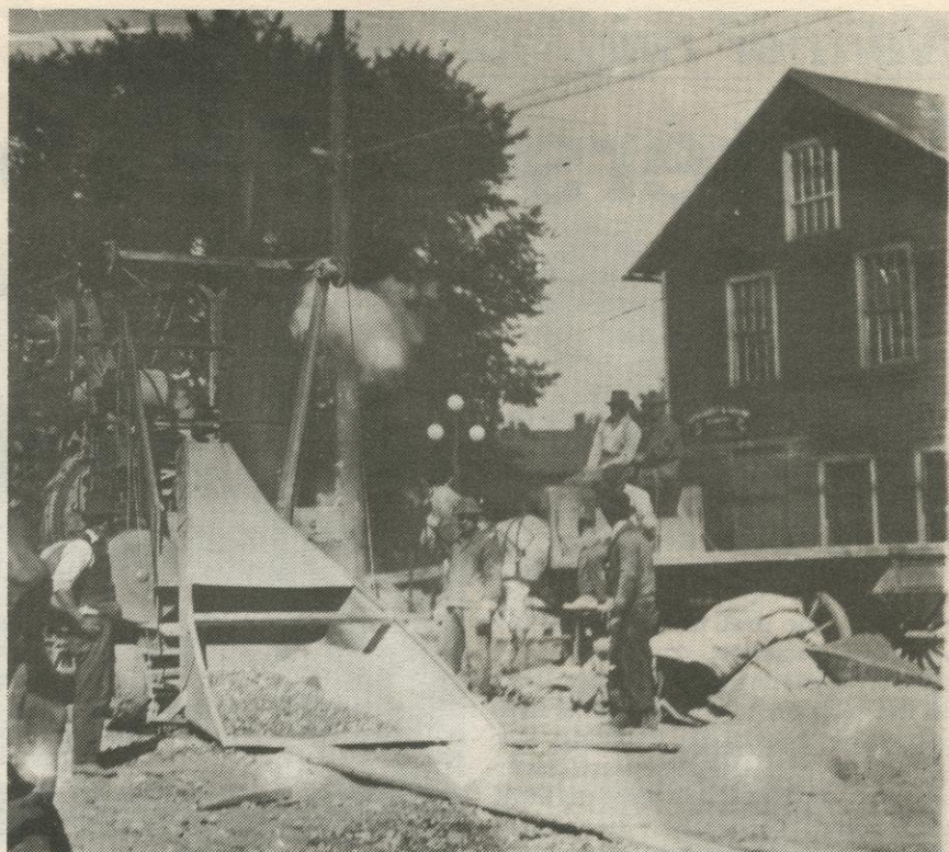
Paving Main Street Fort Atkinson.
