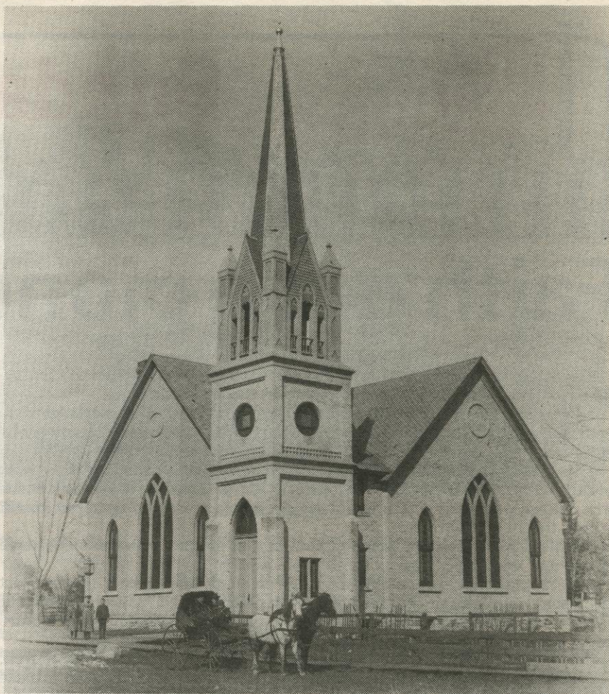
Methodist Church in Fort Atkinson.
