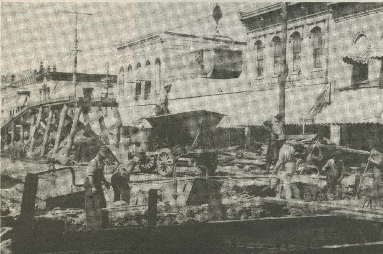
Building Main Street bridge on north side of Rock River.
