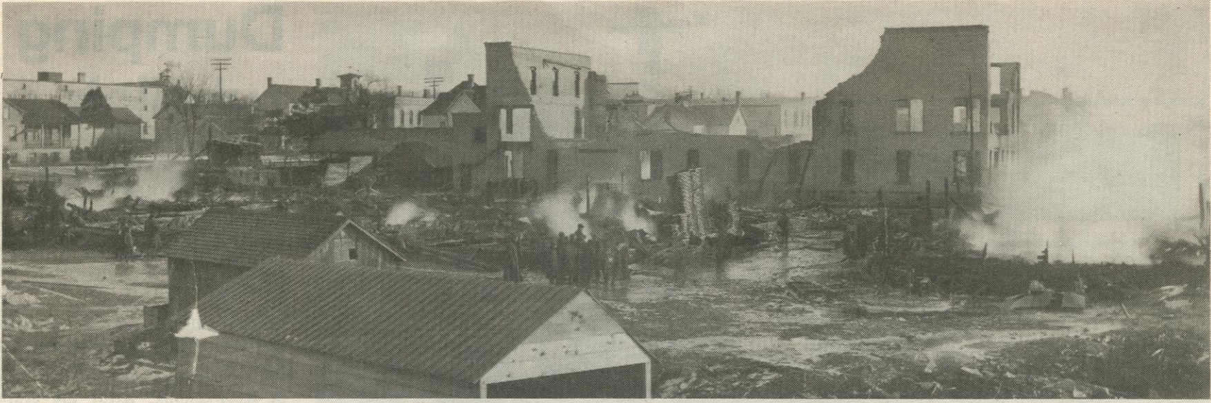
Northwestern Manufacturing burned Jan 6, 1906.
