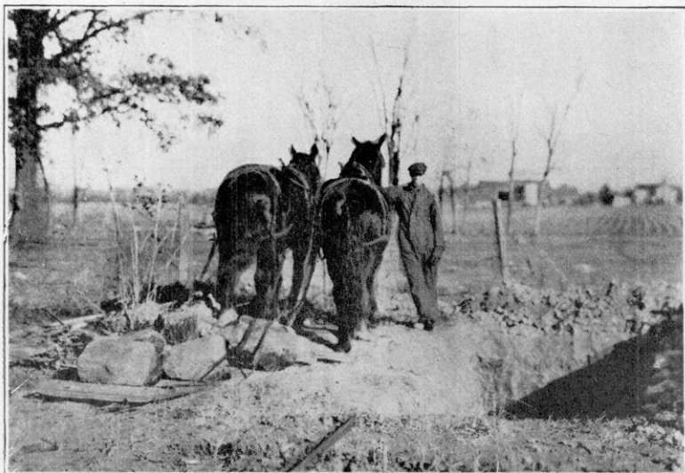
CONSTRUCTING A VERTICAL DRAIN IN A DEPRESSION IN MIAMI CLAY LOAM
