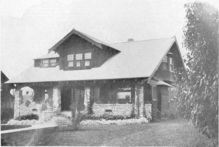
A FORTY-FIVE HUNDRED DOLLAR HOUSE NEAR LOS ANGELES. PORCH ENTIRELY OF COBBLESTONES.
