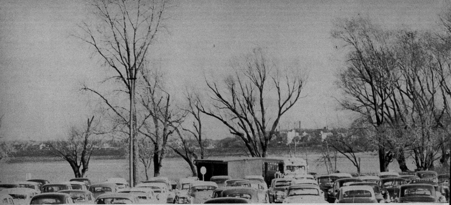
This is "Lot Sixty", which has added hundreds of parking spaces for faculty, staff and students.
