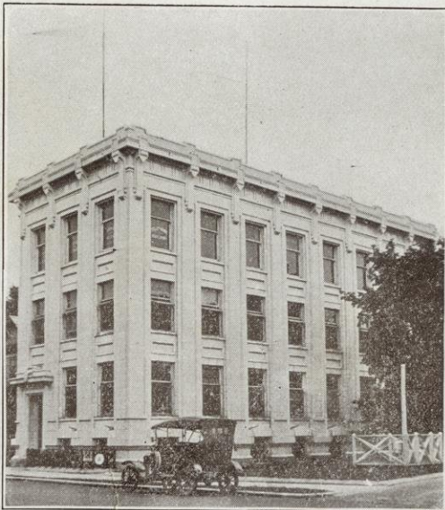
Wausau Telephone Company Building
