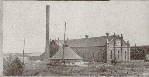
Street Railway System Water Pumping Station
