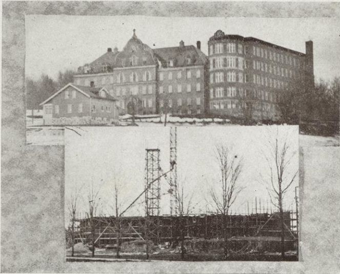
St. Mary's Hospital New Wausau Memorial Hospital (Under Construction)
