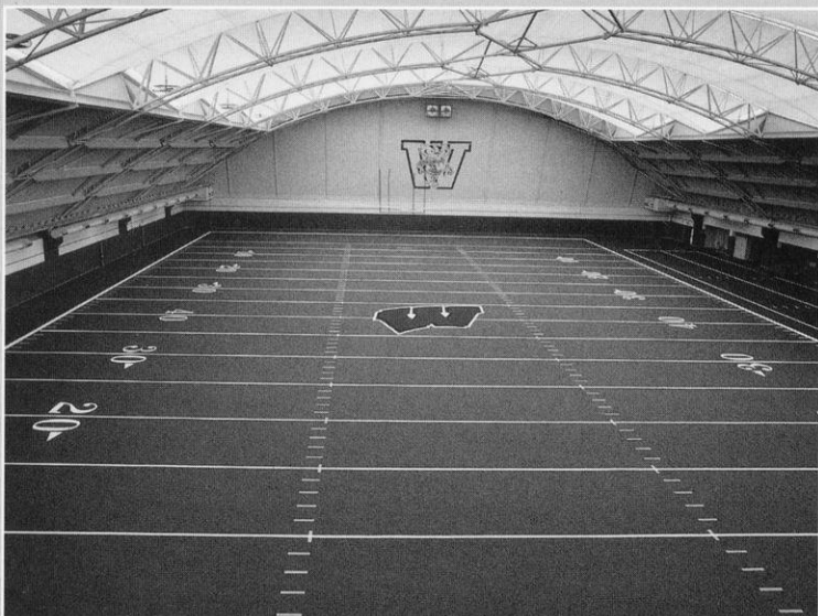
The McClain Athletic Facility features a 90-yard indoor practice field with newly resurfaced artificial turf. The lower level houses the Fetzer Student Academic Center, the headquarters of the Badgers' Sports Medicine staff, a fully-equipped weight room and locker rooms for football, track, softball, and soccer.
