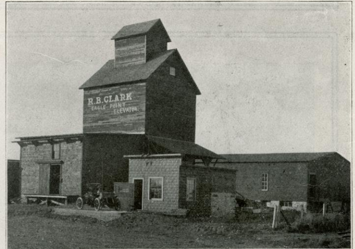
Eagle Point Elevator, Potato and Hay Warehouses
