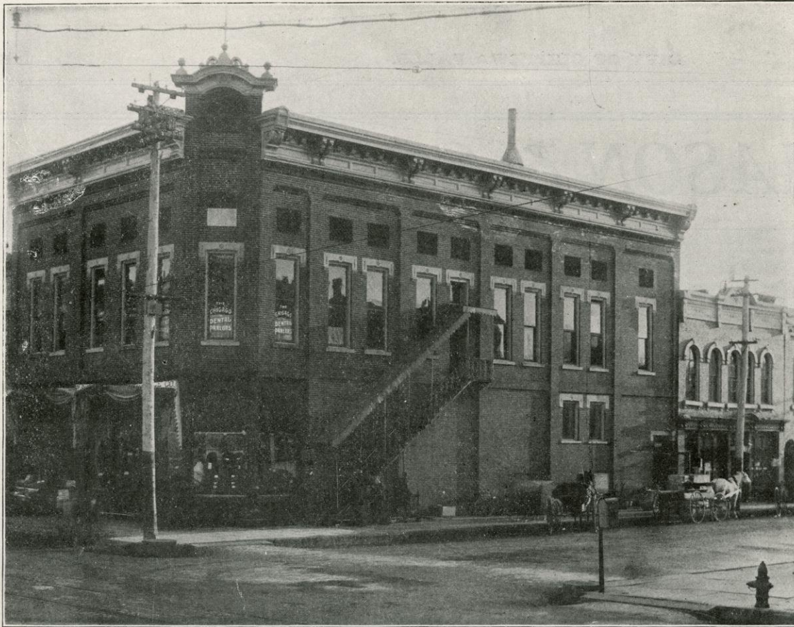
Mandelert Mercantile Department Store
