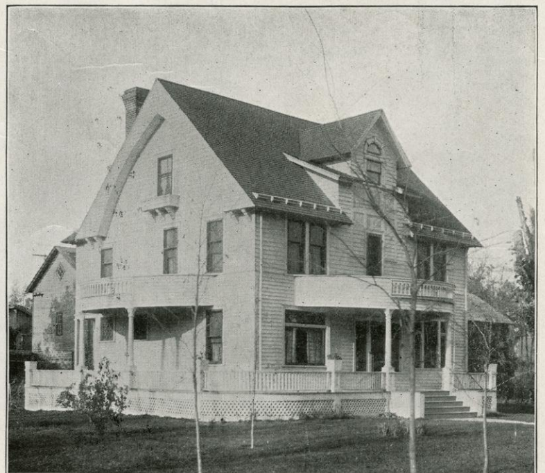
RESIDENCE OF W. S. GREENWOOD.
