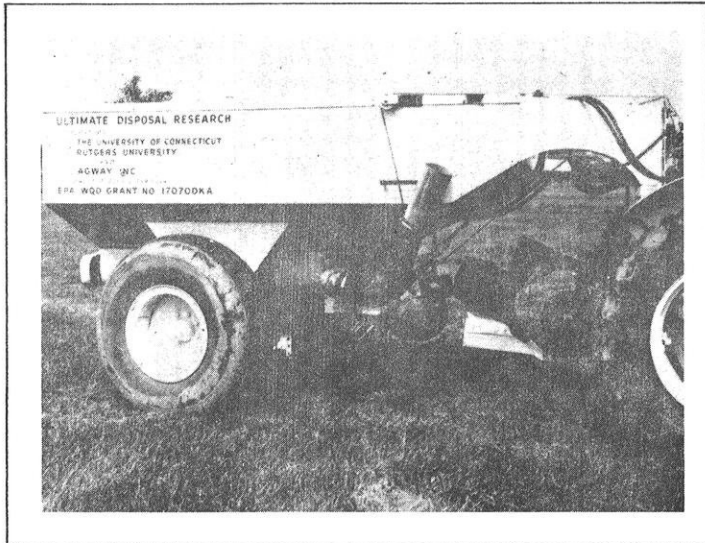
FIGURE 11. Second type of injection plow with 1,000-gal. tank trailer with gooseneck tongue. Injector mounted on three-point hitch of tractor. Courtesy of C.H. Reed, Rutgers University.
