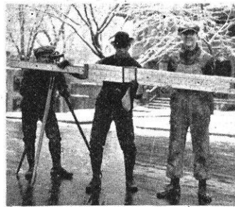
LAYING OUT THE ROUTE
