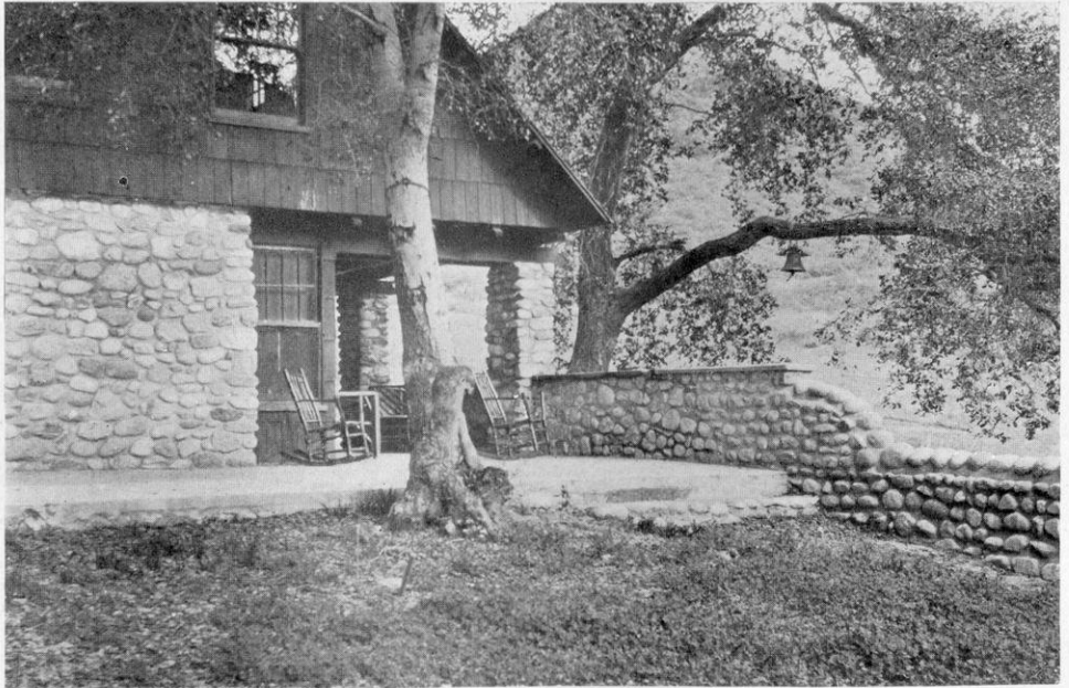
FULL VIEW OF MR. O'MELVENY'S HOUSE, SHOWING USE OF COBBLESTONES IN FOUNDATION WALLS AND GARDEN STEPS.
