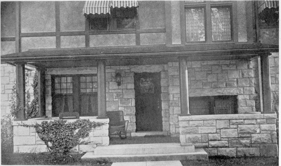
FRONT ELEVATION OF MR. BARBER'S HOUSE IN NORTH ADAMS, MASS., BUILT FROM CRAFTSMAN PLANS.
