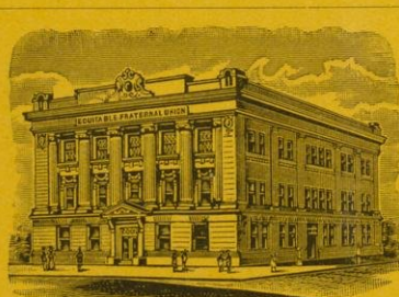
Home Office Building
