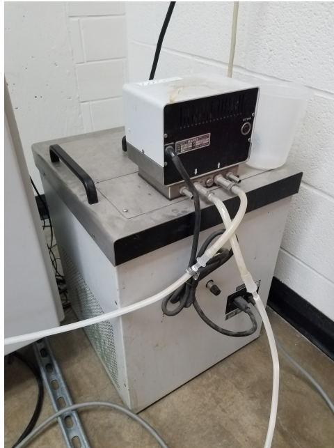
Figure 59: A large recirculating chiller that uses a tubing wrap to maintain the temperature of the ORPs. The chiller is set to a constant 4°C and recirculates constantly when powered by the controller and relay.
