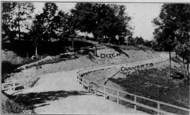
Relocation of the Richland Center—Muscoda road, Town of Richland County. This view shows the proper location of a road to get the best possible grade and provide for the minimum future maintenance cost. The relocation is a seven per cent grade, and the old road directly opposite this point is a fifteen per cent grade. Note the culverts with breaker walls to turn water from the upper ditch and discharge it well away from the road on the lower side. Also note ditch along fence above the upper bank slopes to carry water to culvert rather than down over the slopes.
