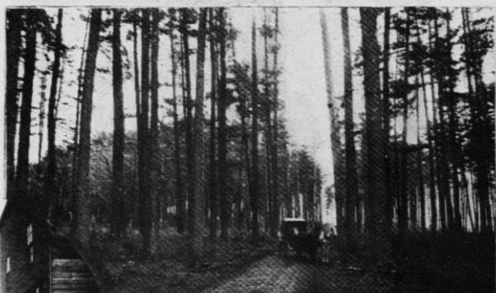
ROAD TO MINONG STATION
