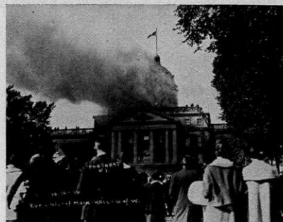
BASCOM HALL: "The dome burned." Students filed from the building in orderly lines and formed volunteer bucket brigades.
