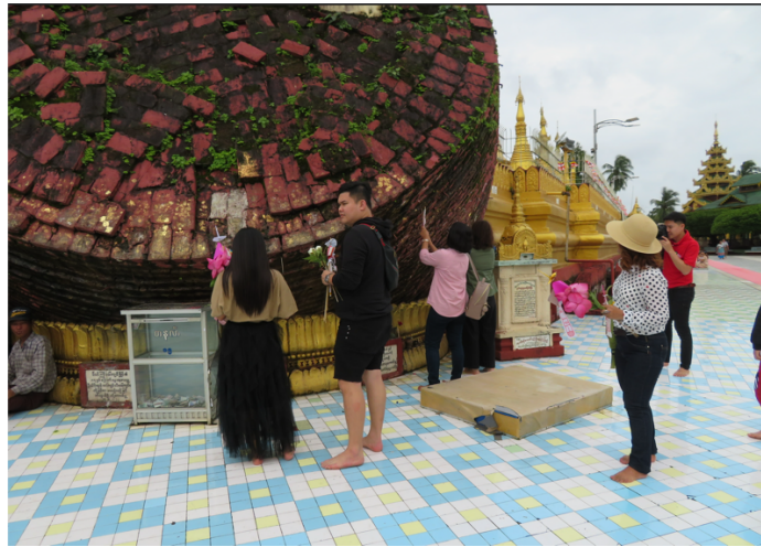
Figure 8. The fallen top part of Shwemawdaw Pagoda.
