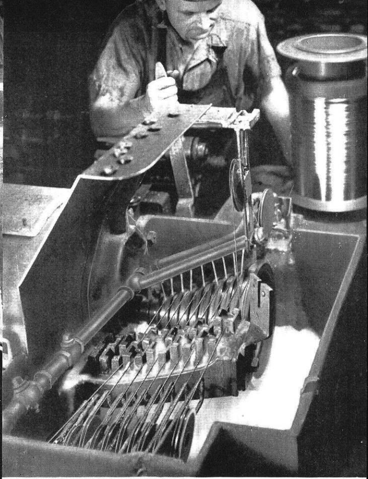
Fig. 22 (Above). Drawing extremely fine stainless steel wire, American Works, American Steel & Wire Co., Cleveland.
