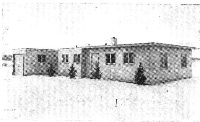
Pre-Fab House Completed
