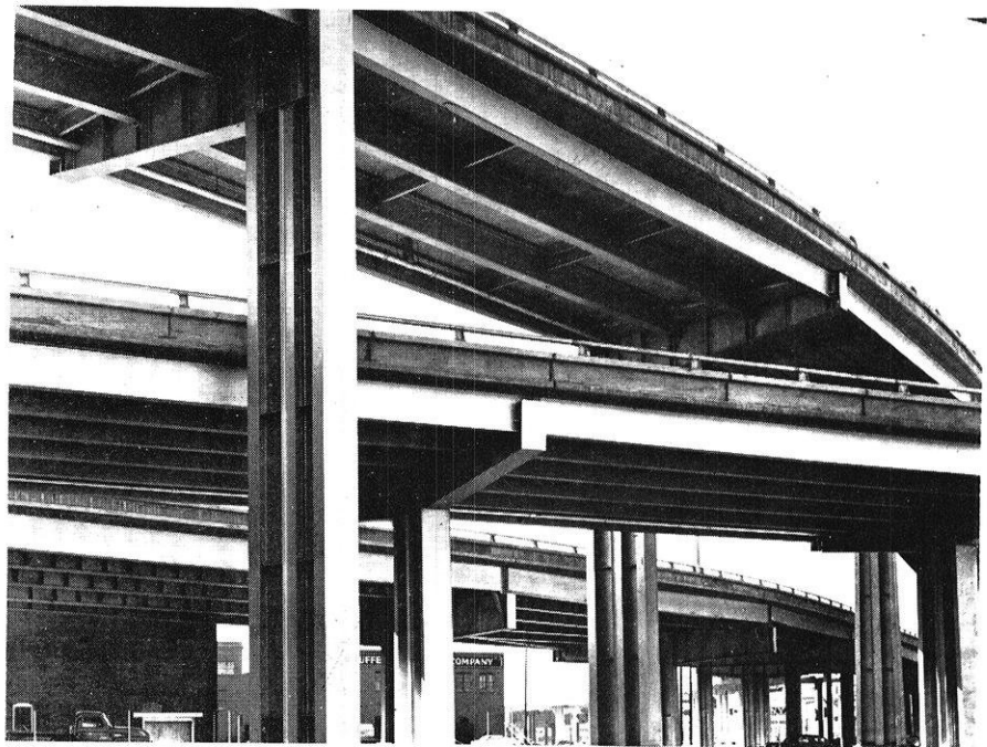
One of the many new welded highway bridges being constructed.
