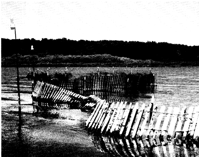
A severe storm with strong winds damaged this wave barrier in Lake Koshkonong. The storm also damaged both the planting of sago pondweed that the barrier was installed to protect and a surrounding natural bed of sago pondweed as well (photo by the author).
