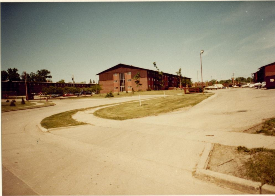
The Hills 3409 South Wollmer West Allis, Wisconsin (2 of 14 buildings)
