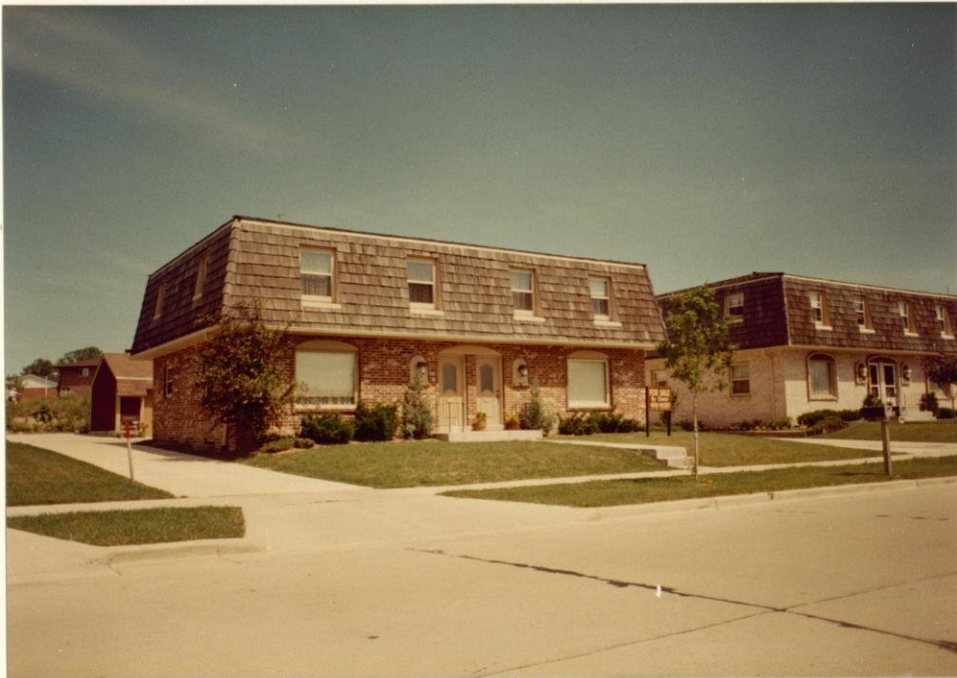
10320 West Grantosa Milwaukee, Wisconsin (adjacent to Wauwatosa, Wisconsin) Build as condo, but rented due to soft condo market
