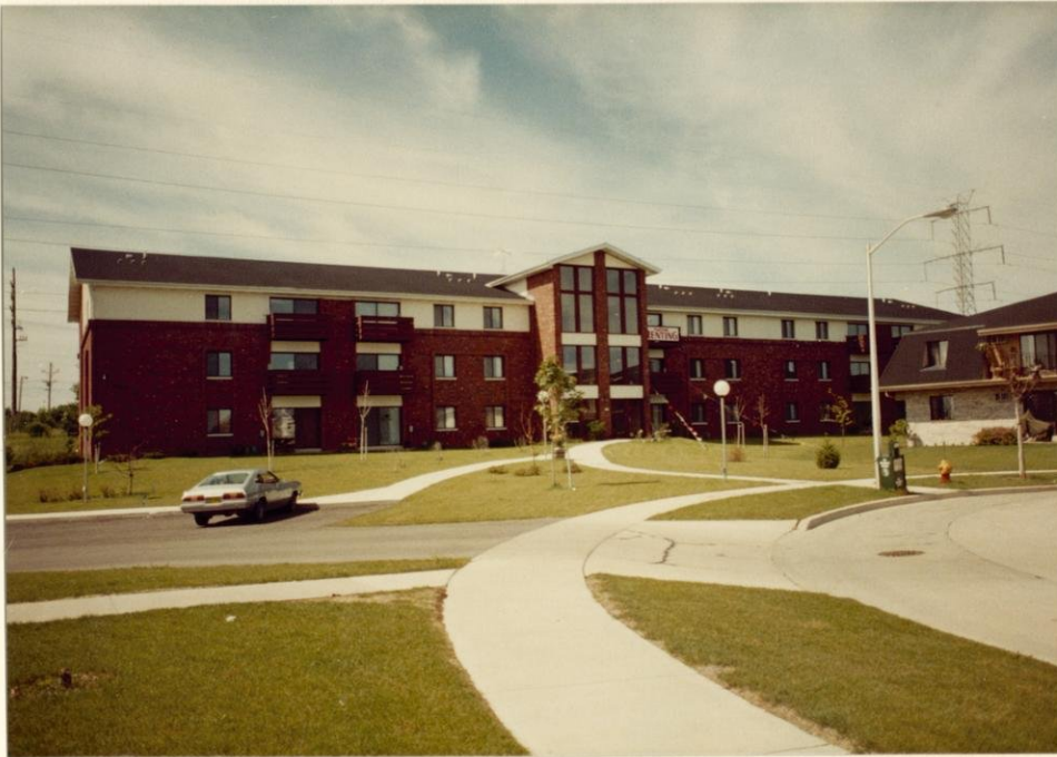
Greenfield Park 1751 South 115th Court West Allis, Wisconsin Built for condo conversion
