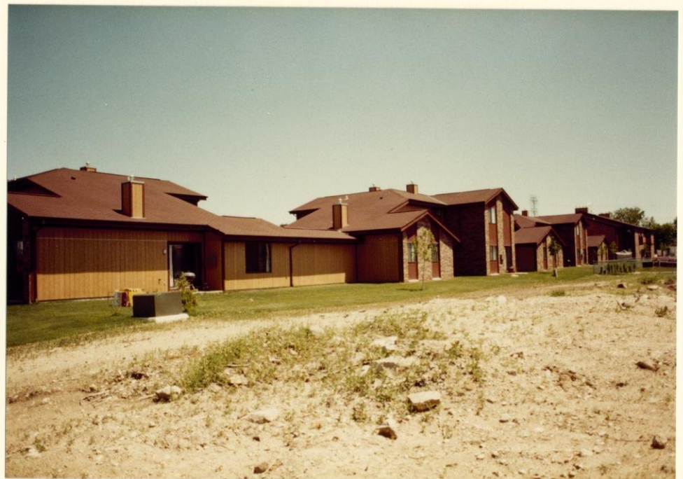
Partial view of the 23 dwelling units connected by common walls located on southern (shown) and western edges of site. Rear yards.
