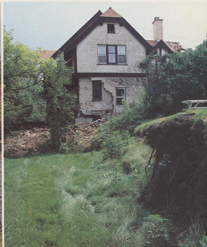
Lakeshore erosion at Whitefish Bay near Milwaukee eats away at a foundation. Photo by Jim Escalante
