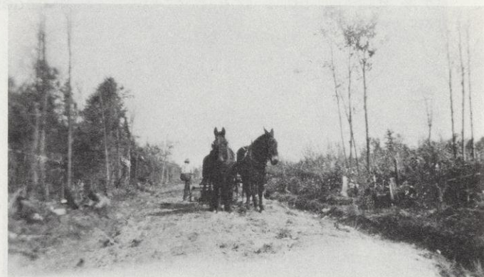
Building the road to Edgewood School
