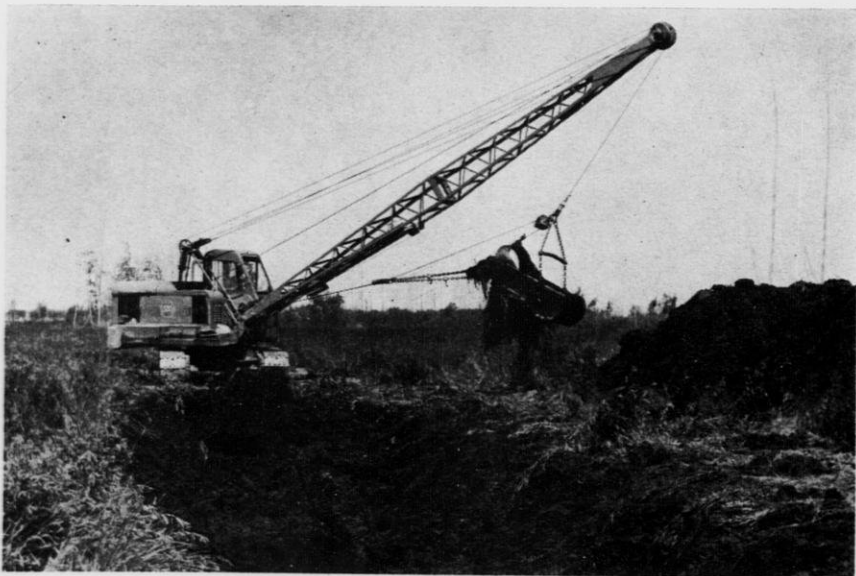
Level ditching creates habitat for muskrats and ducks. Unlike drainage, it leaves marshes wet.
