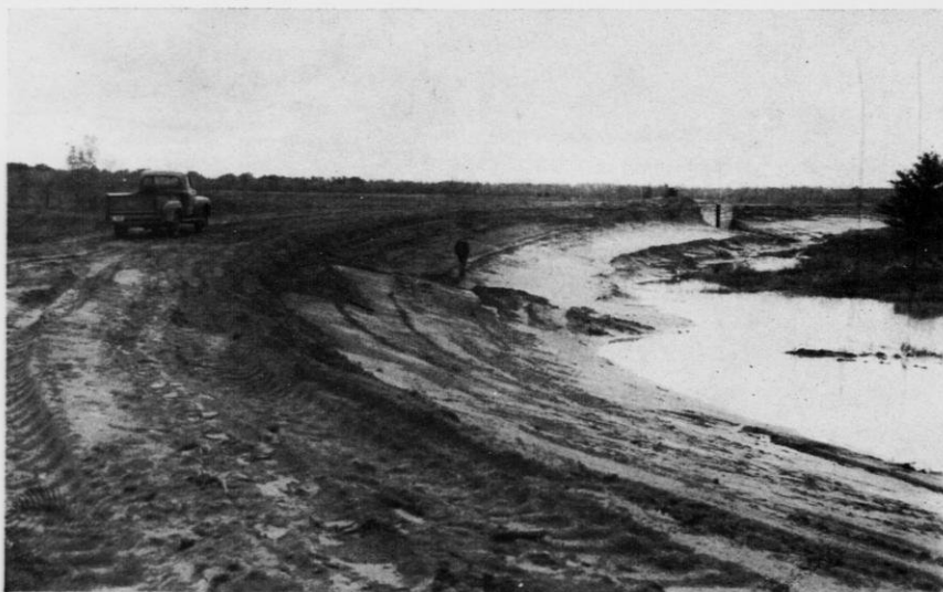
This dike was built to create a wildlife flowage. Large amounts of earth must be moved on such a project.
