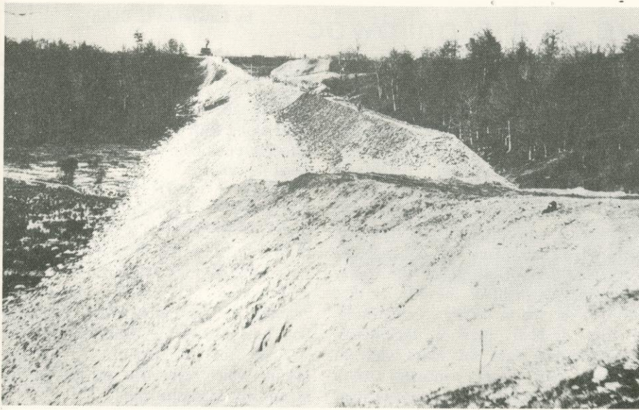
The big cut and fill going into Manitowoc on the Wisconsin Central. The fill area in the center of the photo is just North of Lindbergh Drive.
