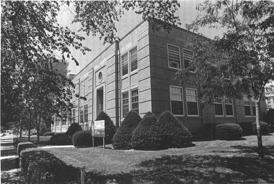
The Highway Lab Building- the center will share it with WCAM (Wisconsin Center for Applied Microelectronics).
