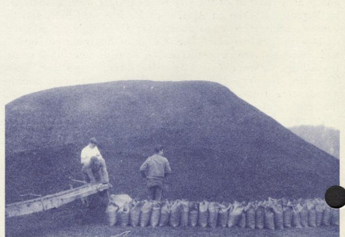
Huge coal pile proved ideal for filling sandbags at Cassville. Conveyer enabled job to be done quickly.
