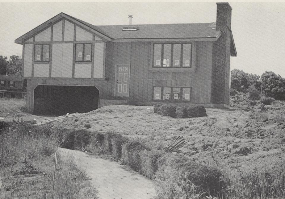
Many builders oppose Madison's comprehensive ordinance which requires control of silt-laden runoff, but city officials say it's working. Here straw bales help check erosion at a local construction site.
