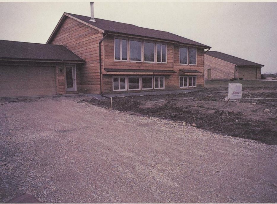
Graveled driveway at a new construction site is good practice.
