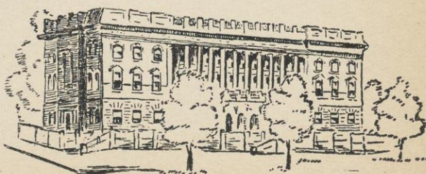
NEW LIBRARY BUILDING.
