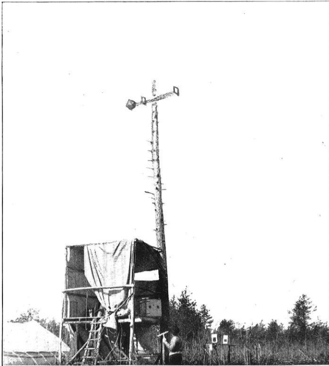
Station Phillips Hill. Showing heliotrope on stub. Elevated to be visible from Station Reid.
