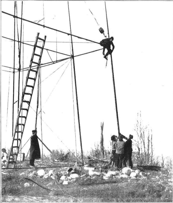
Gaspipe Station during Erection. Entering a Big Leg.
