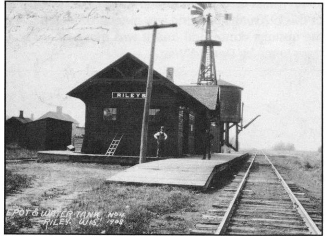
Depot and Water Tank No. 4, Riley Wisconsin, 1908.
