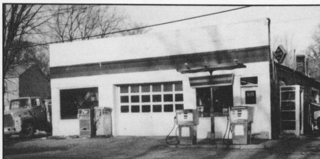
Mt. Vernon Garage and Filling Station.
