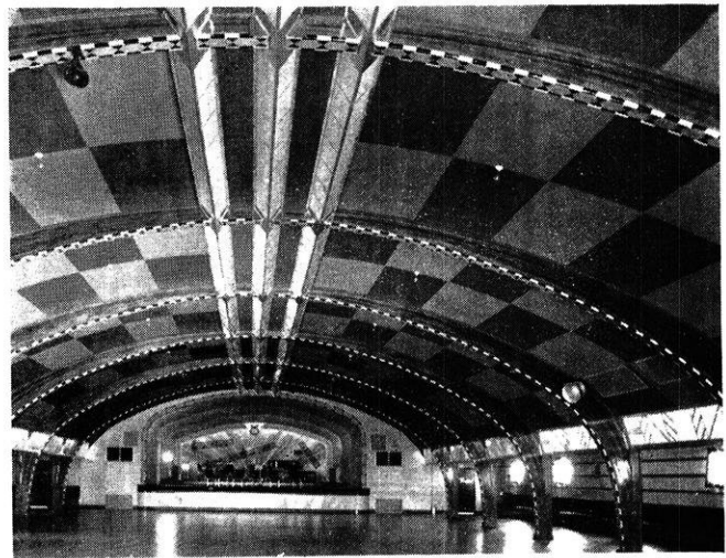
Laminated wood arch construction provides attractive buildings with large unobstructed floor areas.
