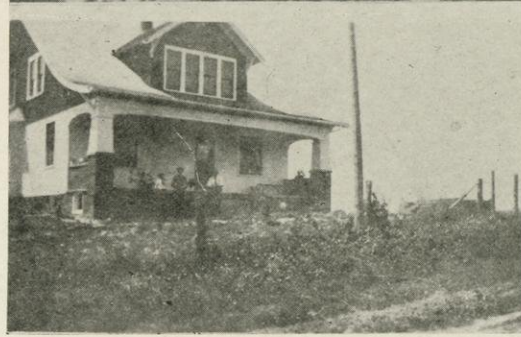
RESIDENCE, BARN AND HENERY OF ROBERT WESENER, R. F. D. No. 1, CLEVELAND, WISCONSIN.
