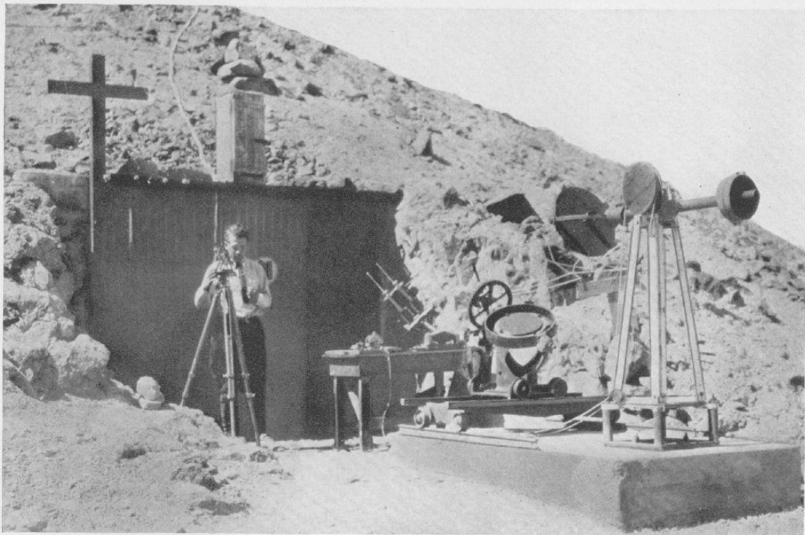
Smithsonian solar station at Montezuma, Chile. An observatory without a telescope where the sun's heat is measured daily
