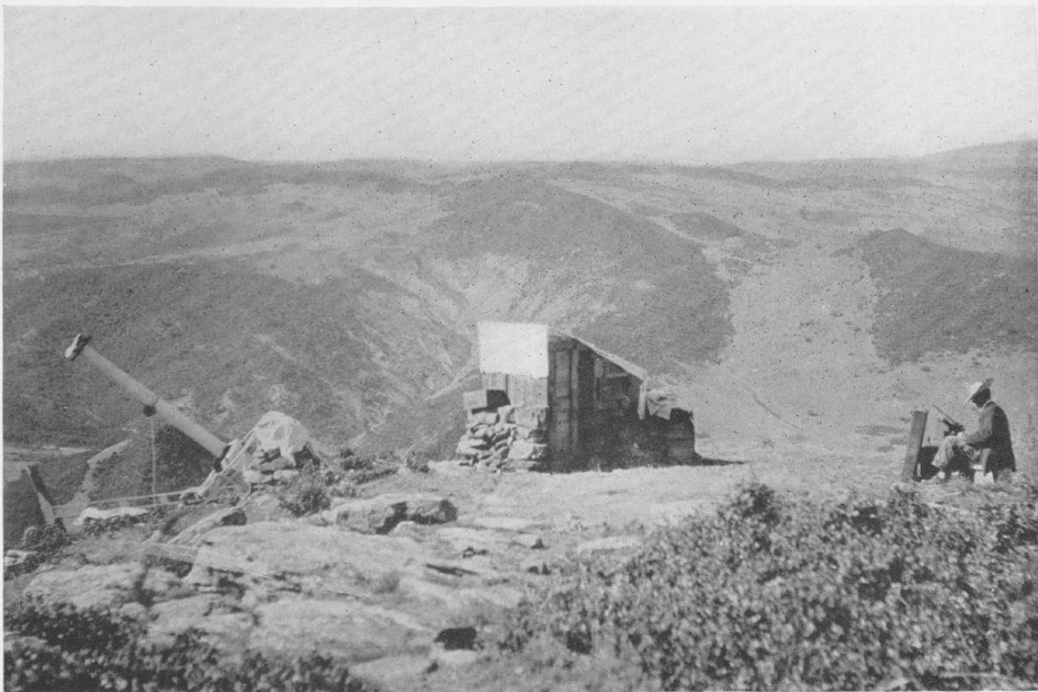
Smithsonian solar-radiation expedition to Bassour, Algeria, 1911. Prof. Brackett observing with the silver-disk pyrheliometer. The instrument shelter is weighted with stones to prevent its being blown away
