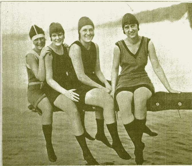
THE FACULTY PIER
