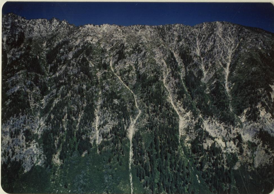
Section 21 10 (G29): Looking North at South Face of Slope
