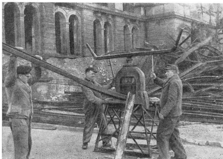
Iron girders, salvaged from the ruins of bombed German buildings, are straightened by workers with a spindle press. The girders will be used in the construction of new buildings.
