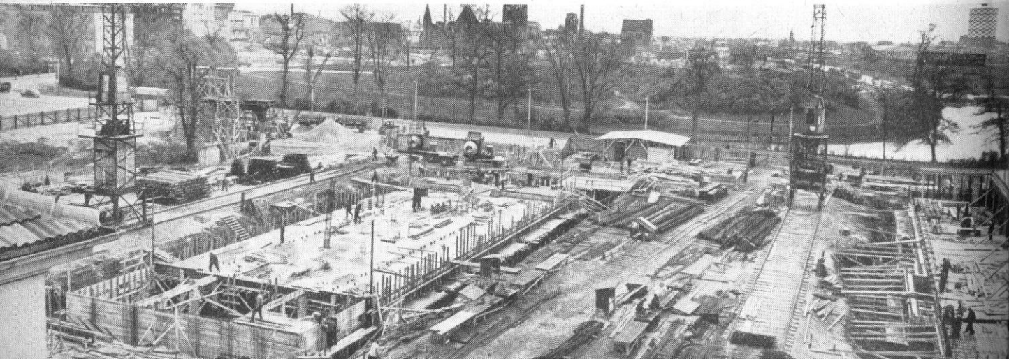
View of foundation construction at site of the new center.
