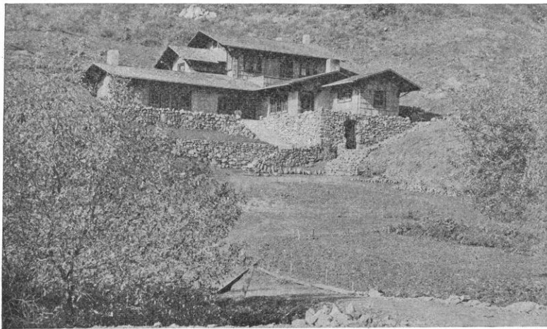
HOUSE IN RELATION TO HILLSIDE: DESIGNED AND BUILT BY A. R. KELLY.
