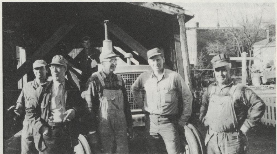
Moving a shed
