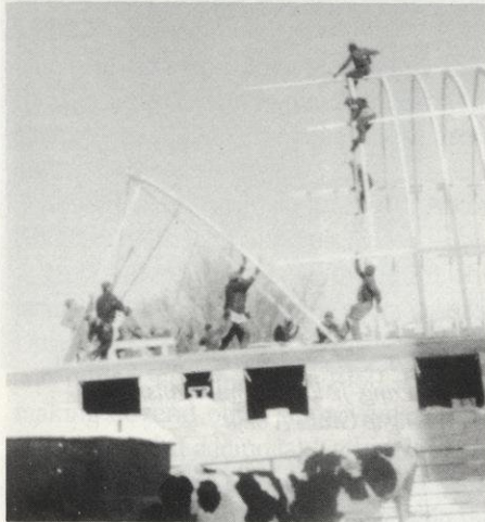
Friends and neighbors rebuilding barn
