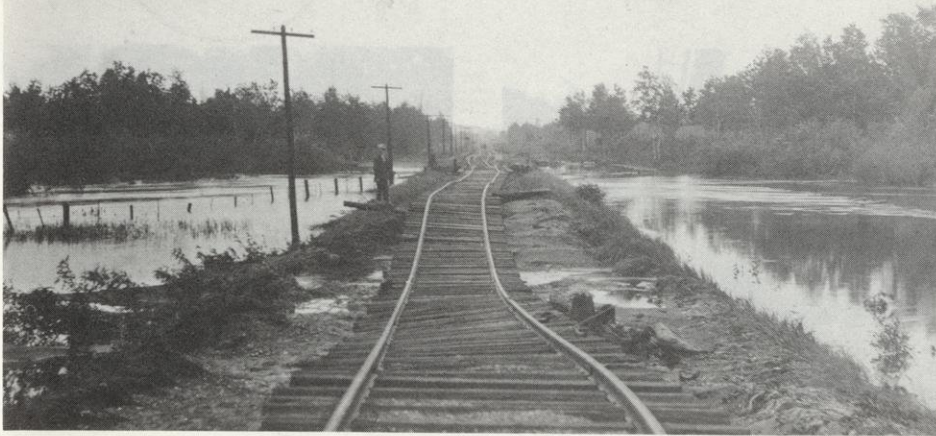
Wash out of C & NW tracks 3/4 mile long near Edgar - 1914
