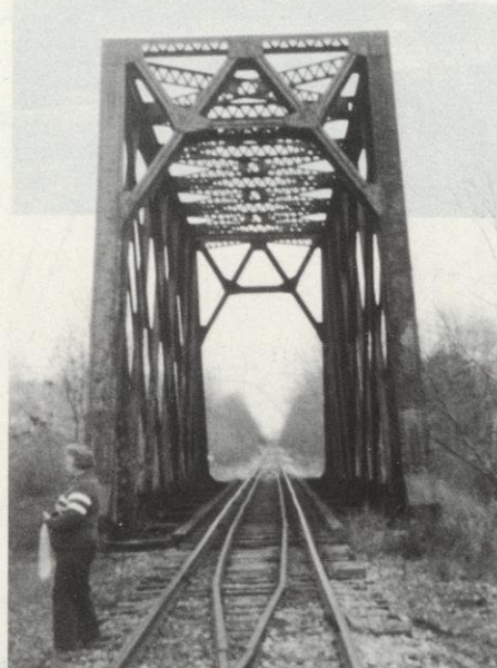
Railroad Bridge-courtesy of John A. Koppa
