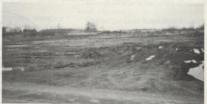
Cassel town hall building site from Hwy "S"
