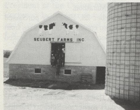
Another barn addition completed
