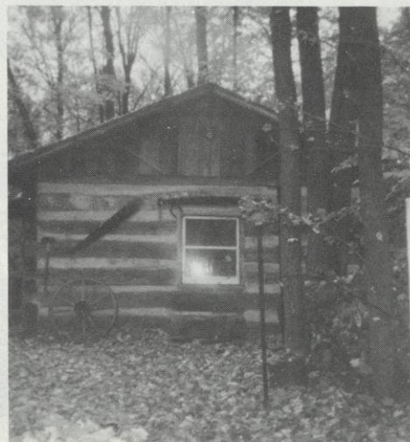
Cabin rebuilt on the Lang farm - 118 years old
