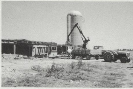
tearing down barn
