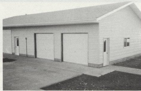
Drying shed and garage built in 1987, destroyed in May 1988 tornado and rebuilt identically in August of 1988
